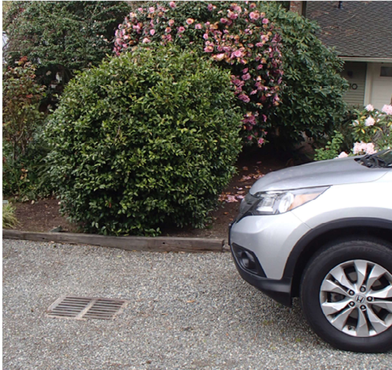
Photo No. 5 Looking east at CB 30a-24 at House #6110.
