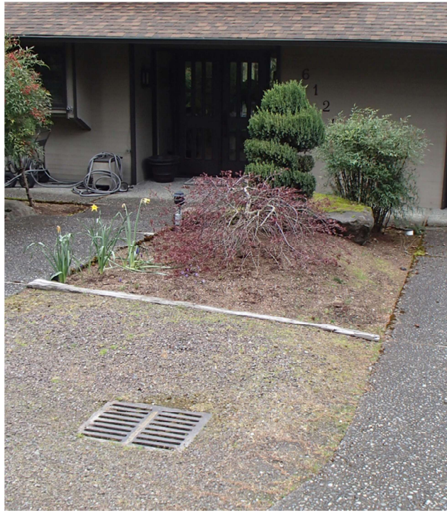
Photo No. 4 Looking easterly at CB 30a-11 in front of House #6120.
